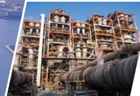
From top: Coal reclaimer; torrefied pellets, which simplify handling of biomass through low-temperature carbonization; waste plastic processing plant; kiln at Kyushu Plant
