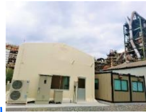
Methanation Test Facility
