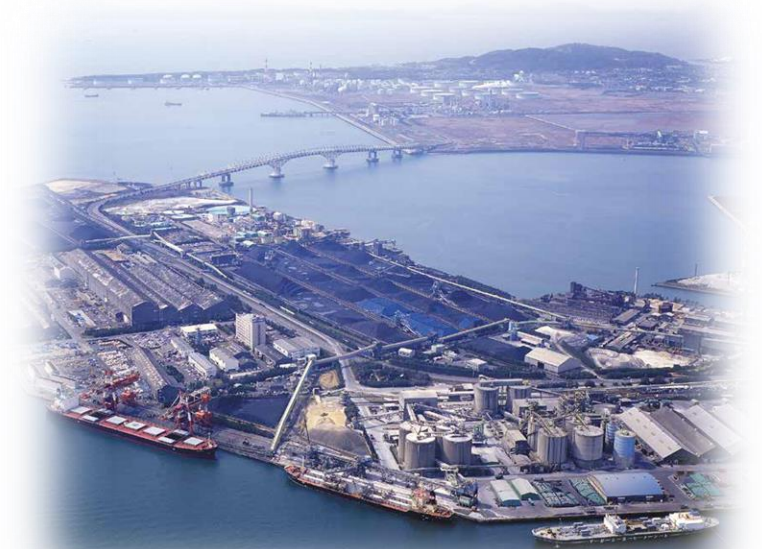
Ube Cement Plant & Ube Coal Center
